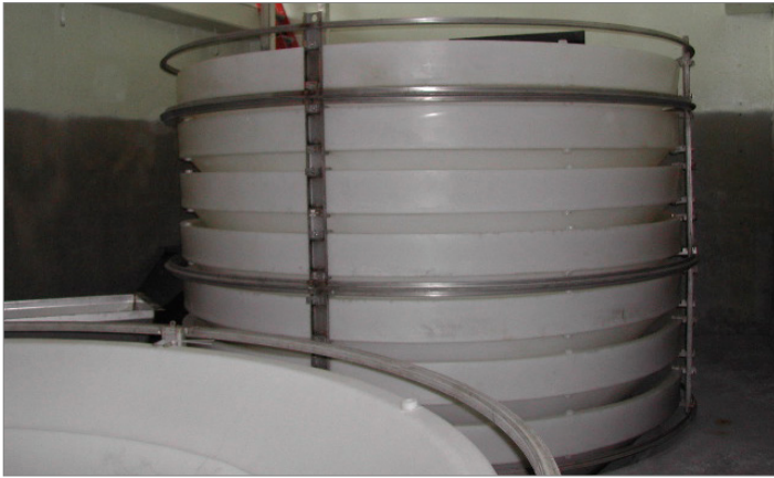
HeadCell® Units Retrofitted into an Aerated Grit Basin at the Council Bluffs, IA Plant
